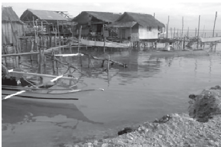
Zamboanga: The village will get sanitation and clean water installations.
